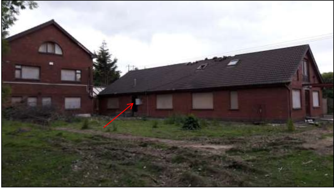
Plate 22. House 3 in 2018 - long extension building which contained the boiler house (indicated by the red arrow).
