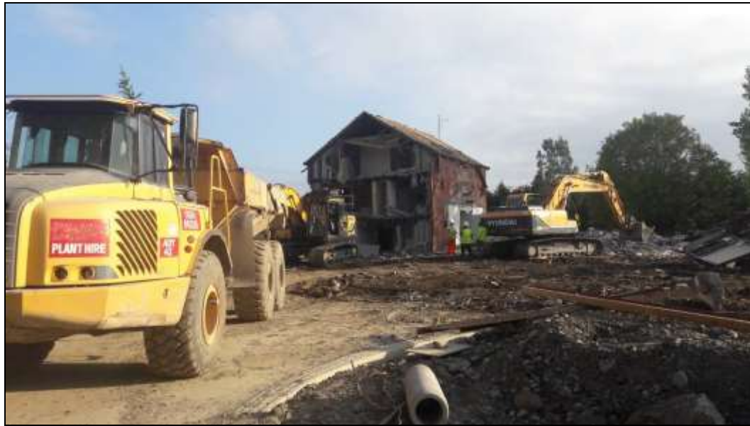
Plate 30. Demolition of the easternmost house in October 2018.
