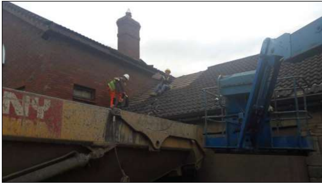
Plate 26. Roof stripping of the easternmost house in October 2018.
