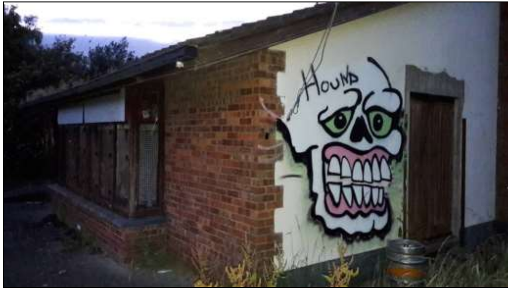
Plate 25. Former rugby clubhouse building in 2018.
