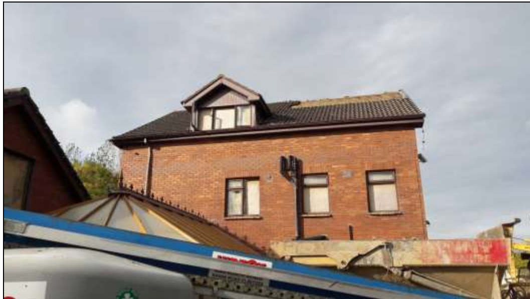
Plate 29. Roof stripping of the easternmost house in October 2018.
